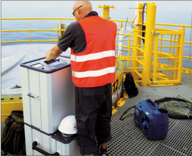
VLF CR-60 kV in operation on the "Baltic 1" wind park (Baltic sea).
